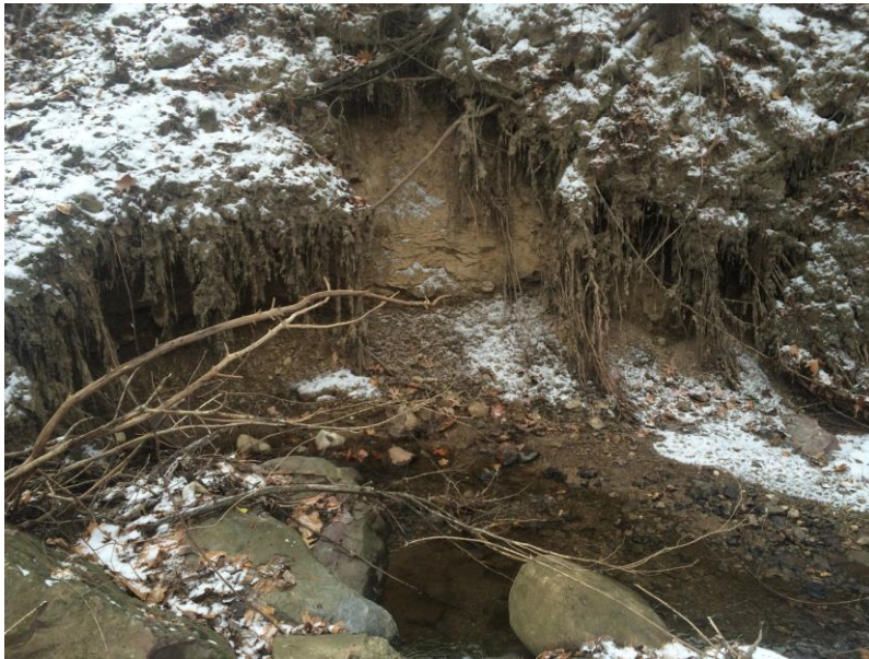
Figure 4: Streambank erosion and incision in Farrell Brook
